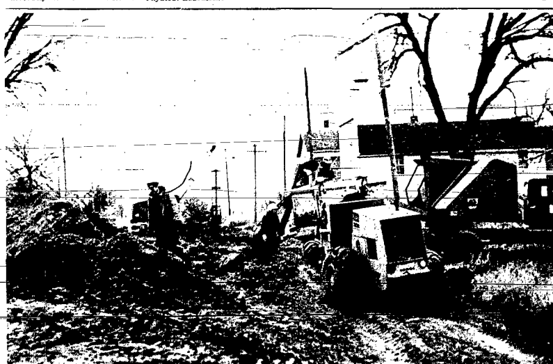
Filling trenches for Dixon Sewer System.
